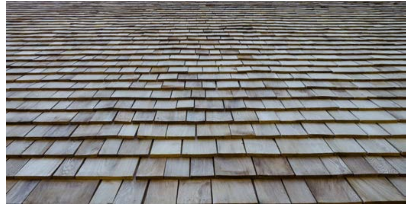
EXTERIOR ROOFING DIRECTION (White Cedar Shake)
