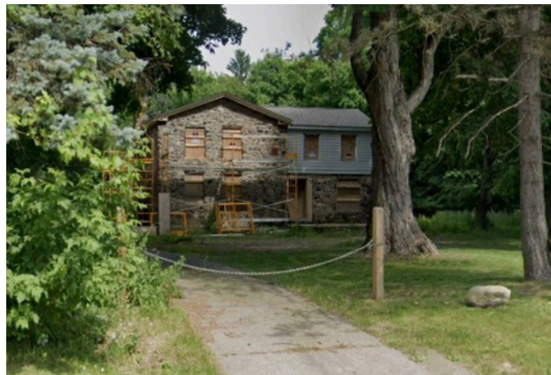
LORNA STONE HOUSE - EXISTING VIEW FROM S. ADAMS RD.
