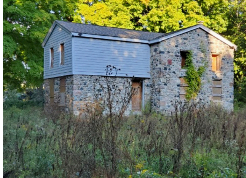
LORNA STONE HOUSE - EXISTING VIEW FROM SE
