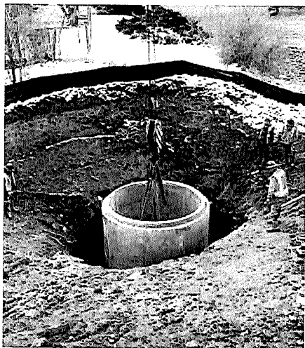
Step 1: Install the base section.
