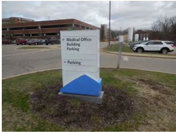
Existing 4'-9" x 2'-6" sign to be removed & replaced; Install far enough away to avoid existing footer
