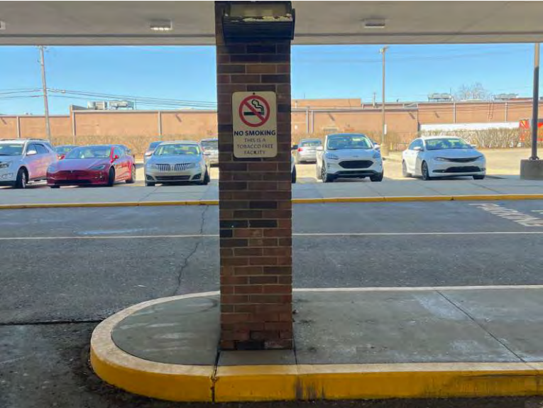
Existing 1'-6" x 12" panel to be removed & replaced. Fill holes w/ matching caulking
