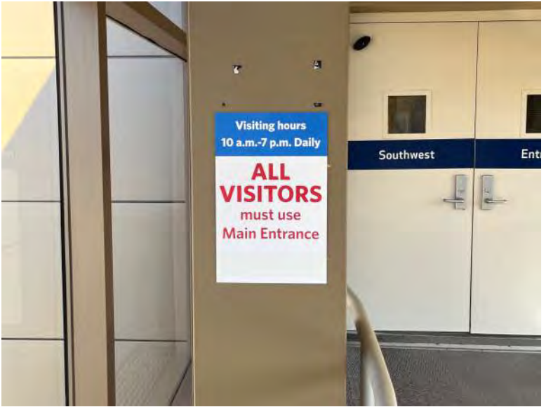
Existing 1'-5" x 11" signage to be removed & replaced; Fill holes w/ matching caulking
