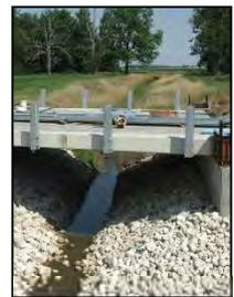
Figure 2: Slab bridge
