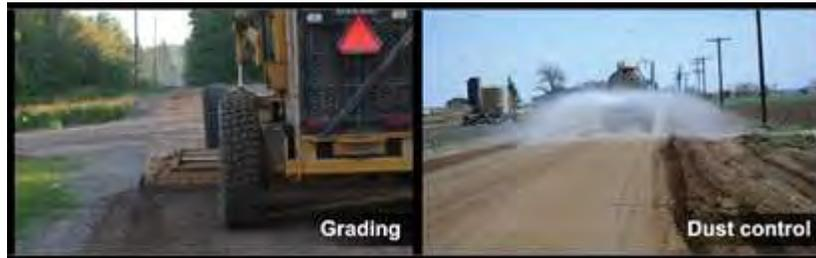
Figure 6: Examples of capital preventative maintenance treatments cont'd (left) gravel road undergoing maintenance grading, (right) gravel road receiving dust control application (dust control photo courtesy of Weld County, Colorado, weldgov.com)
