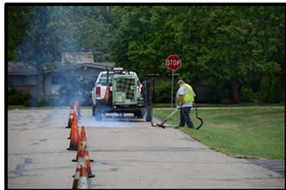
Figure 5: Example of crack sealing capital preventative maintenance
