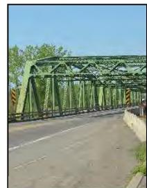
Figure 3: Truss bridge
