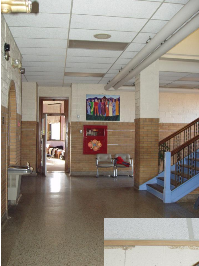
Photo 6: Main first floor corridor in 1929 building.
