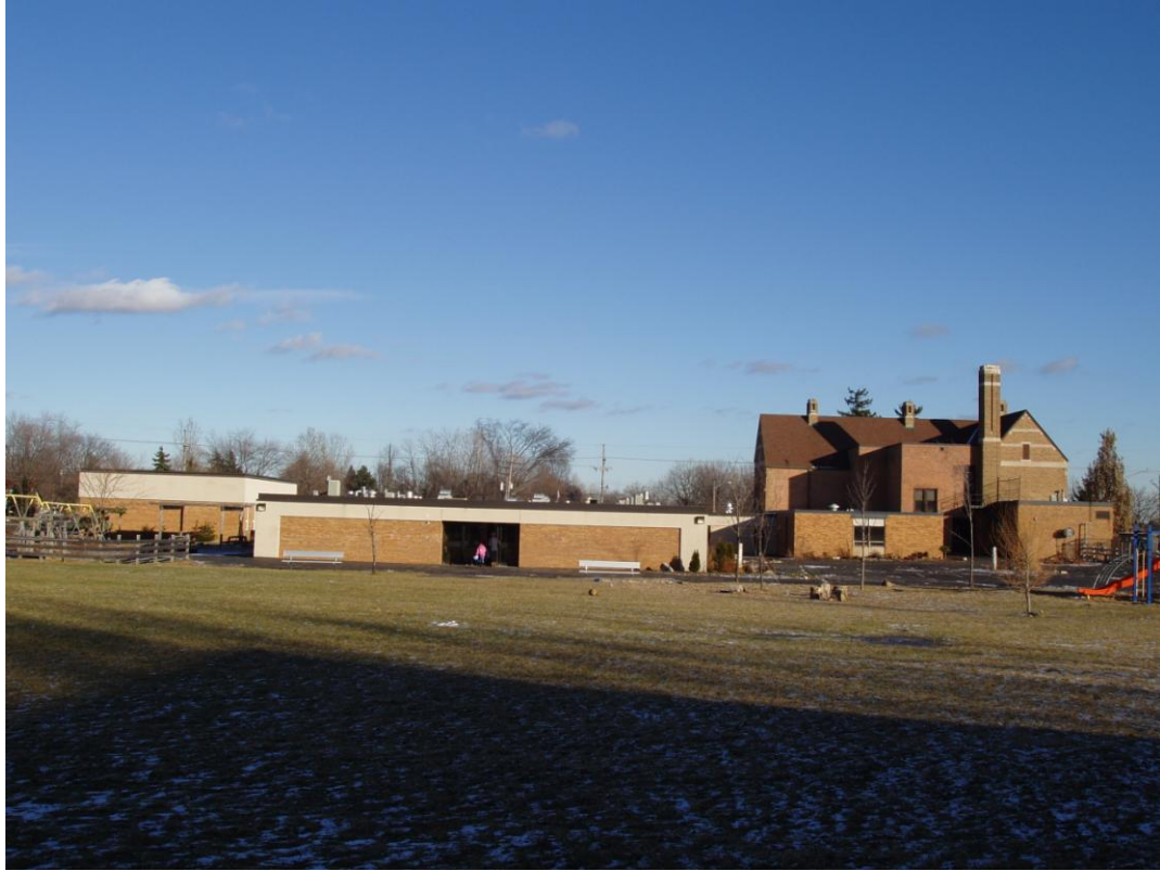
Photo 2: South elevation, note first floor bay for kindergarten room.
