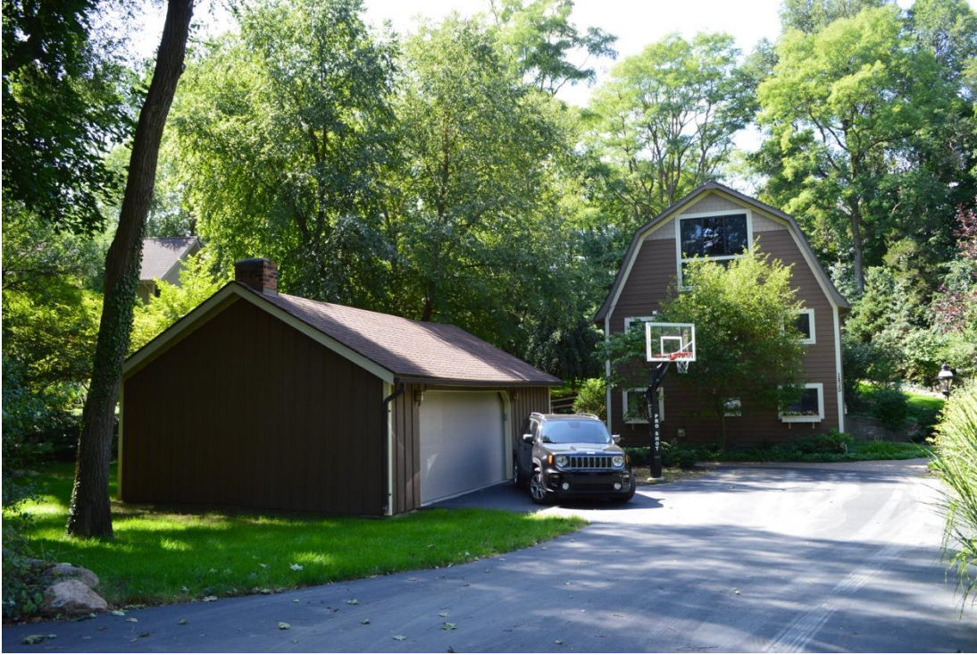
1820 Carter, barn converted to a house, non-contributing
