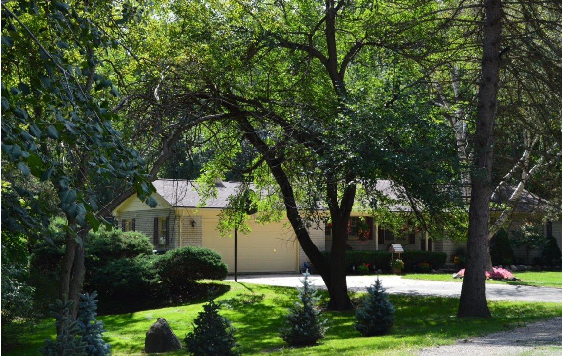
1650 Washington Road, 1964, non-contributing
