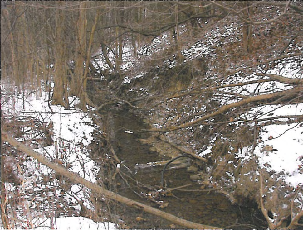
3. View of exposed utilities and one of several hillslope failures – facing downstream (R. Hills)
