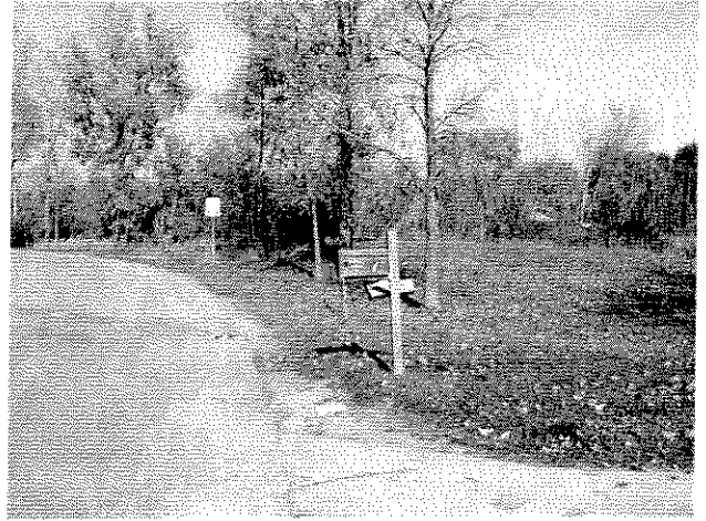
Looking north northwest along Hazelton Avenue.
