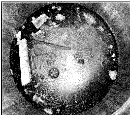
Floatable debris in the Aqua-Swirl®
