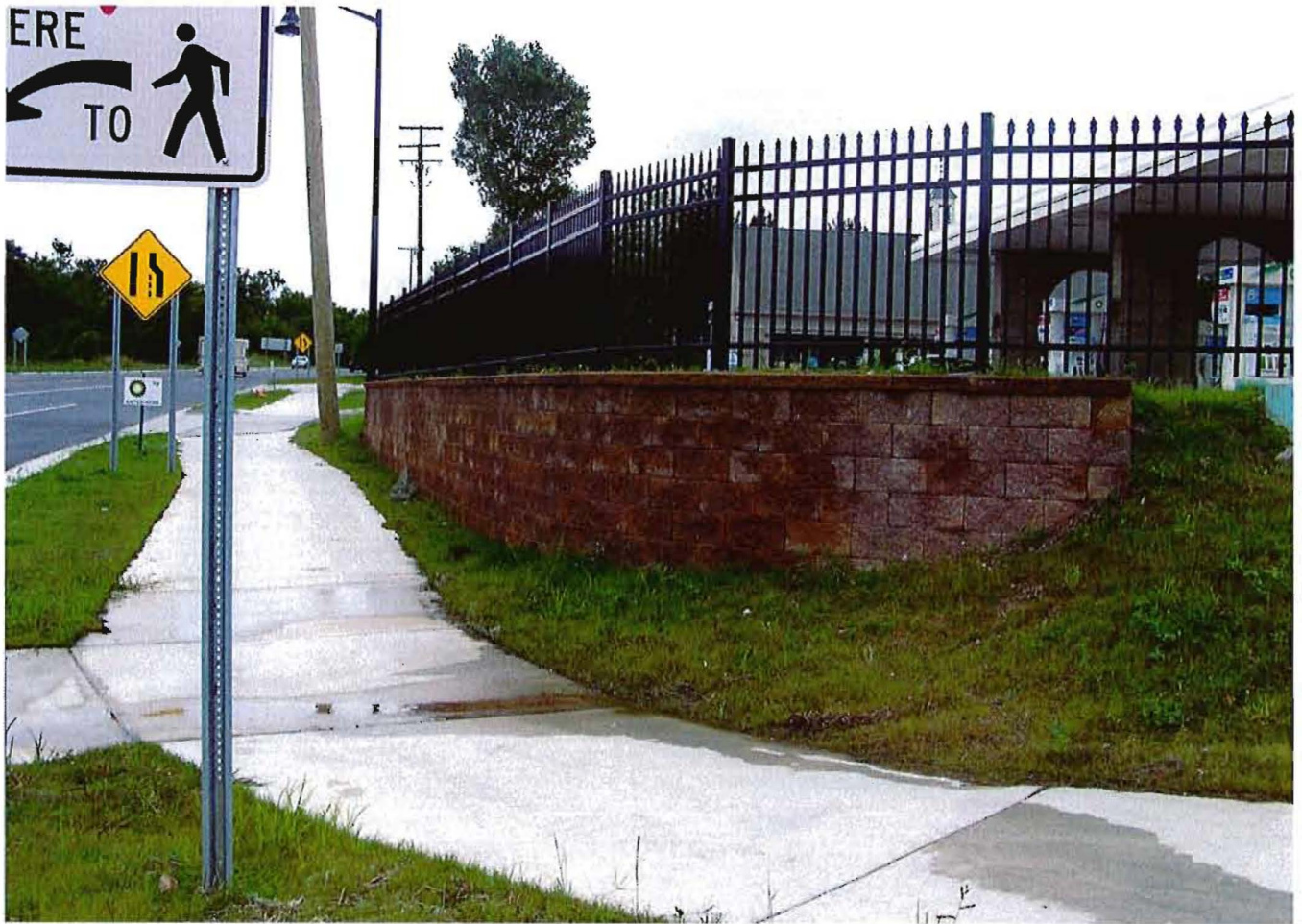
PHOTO #7 - RETAINING WALL - 14/FARMINGTON Rd
