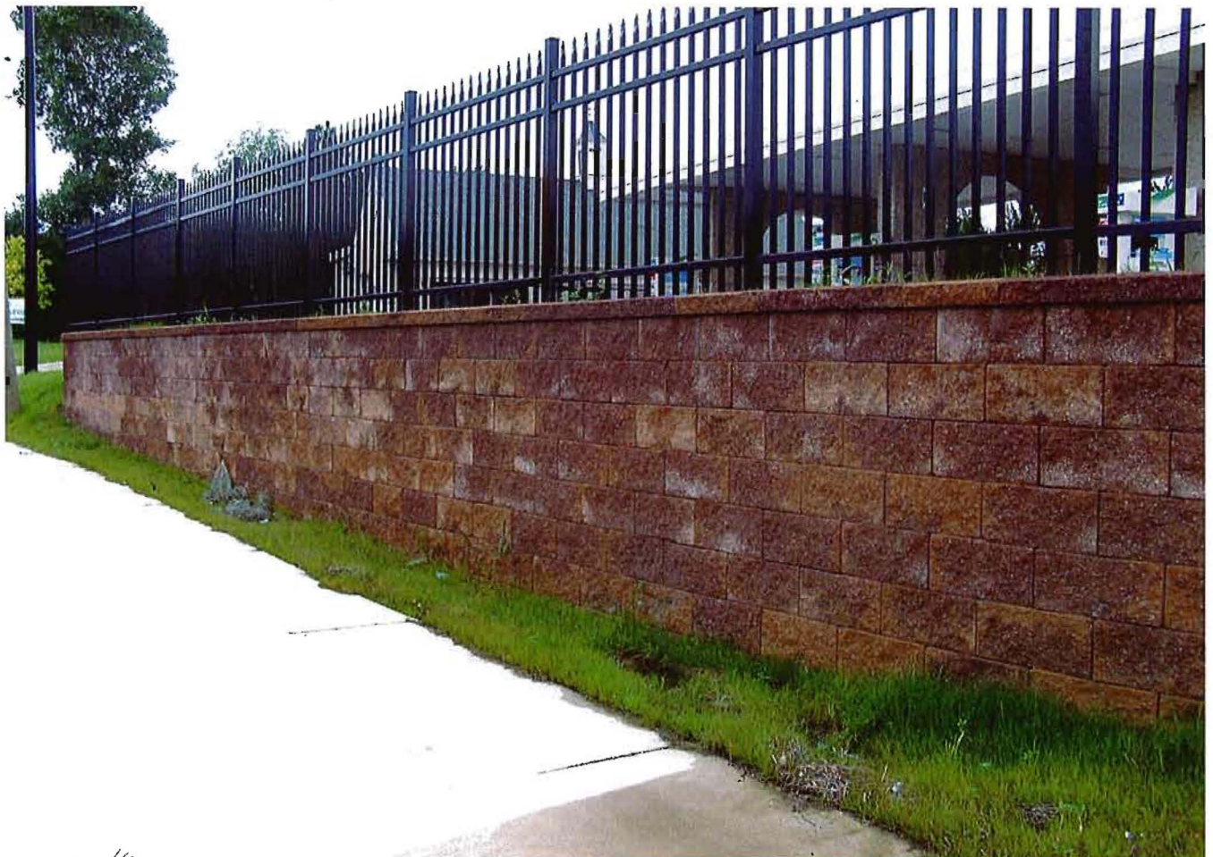
PHOTO #8 - RETAINING WALL - 14/FARMINGTON Rd
