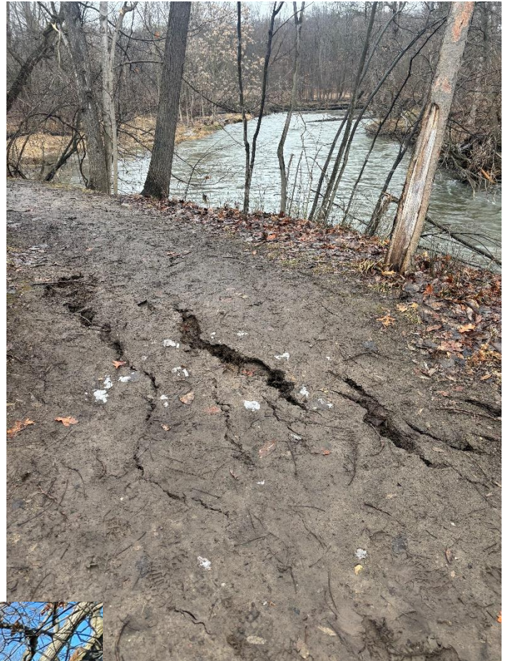
Photo 2: Turtle Trail Bank Failure – Looking upstream,
