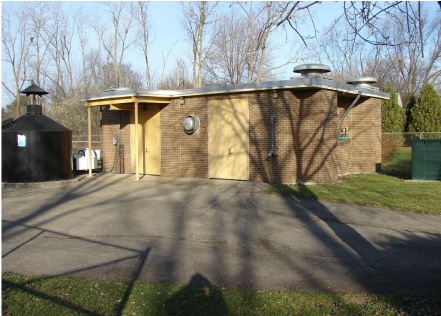
Existing Grant Pump Station
