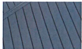
Standing Seam Metal MANUFACTURER: PAC-CLAD TYPE: SNAP-ON STANDING SEAM PANEL SIZE: 12\" O.C. PANEL - 1\" HIGH FINISH: PRE-FINISHED ALUMINUM COLOR: CHARCOAL
