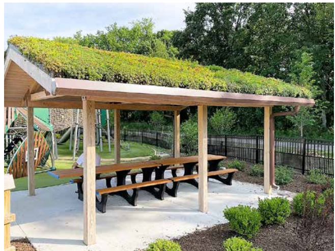
Green Pavilion Picnic Shelter
