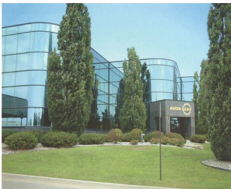
Avon Gear building at 2770 Research Dr., Rochester Hills
