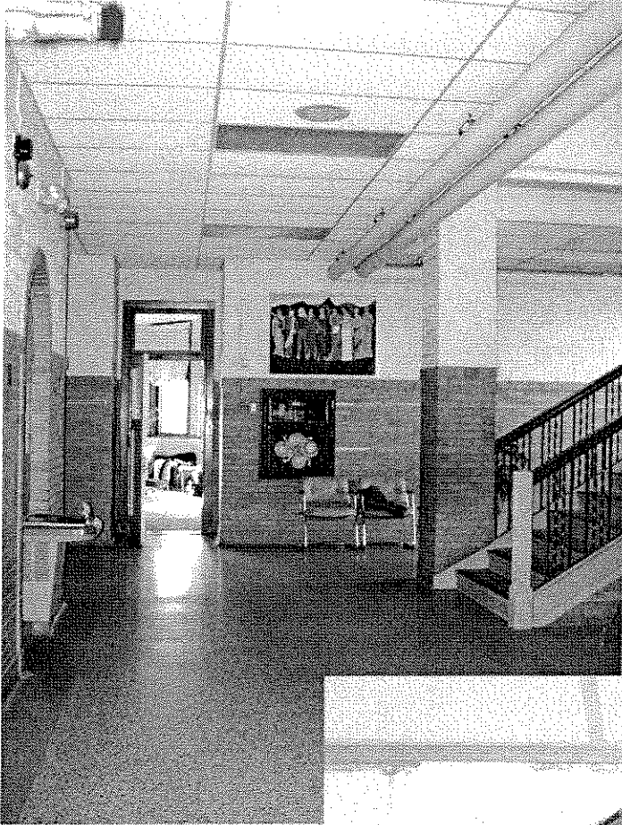
Photo 6: Main first floor corridor in 1929 building.
