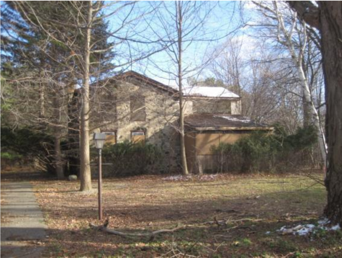
View of the front of the house, looking east
