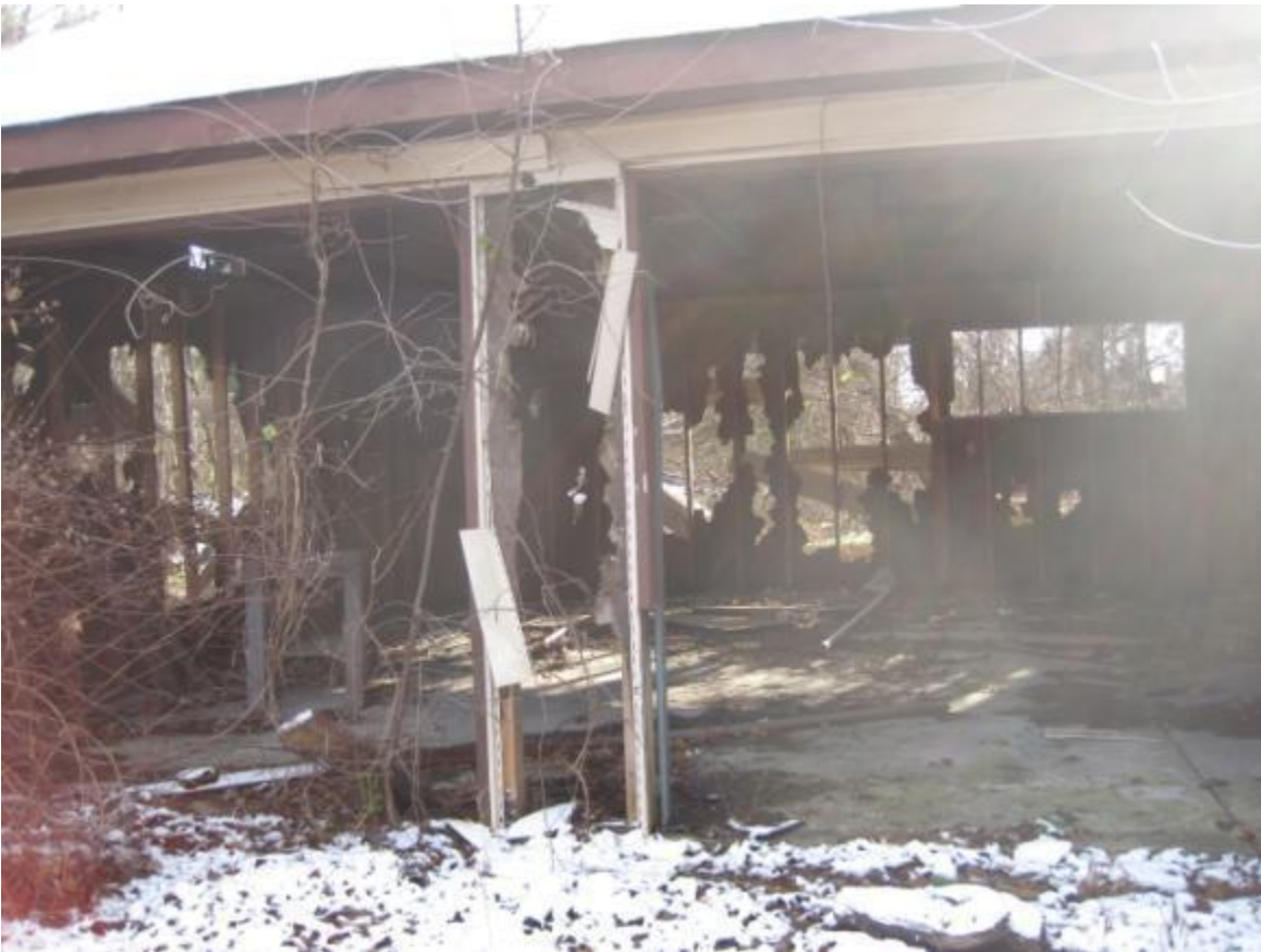
Detail of garage looking south
