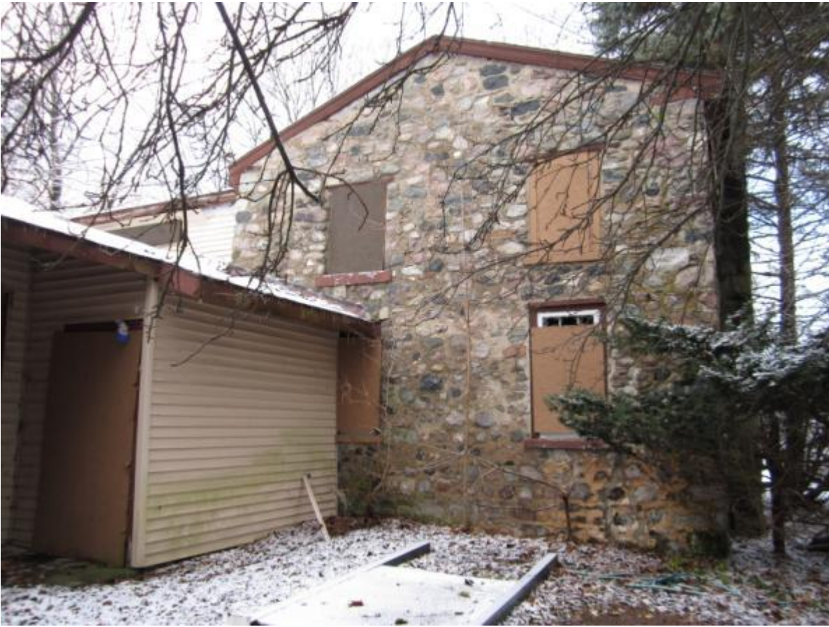
Detail of rear of house, looking west
