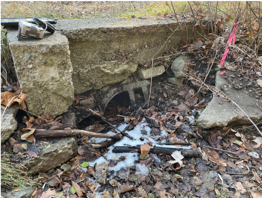
12 – Dual culverts under existing drive, facing southwest
