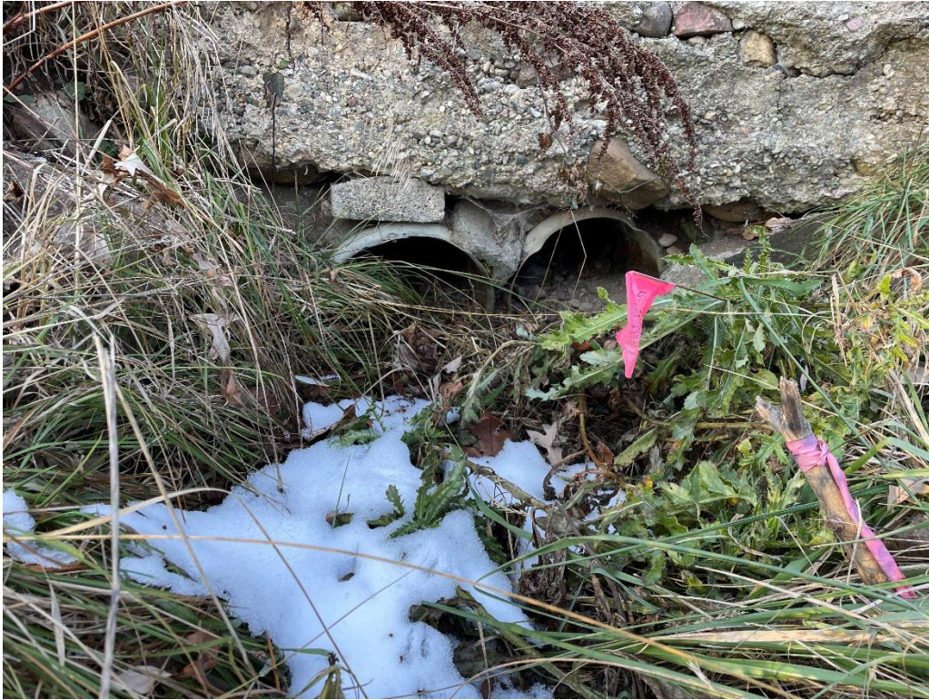
14 – Dual culverts under existing drive, facing north
