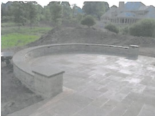
Overlook, Sitting Area and Main Terrace Paving Materials
