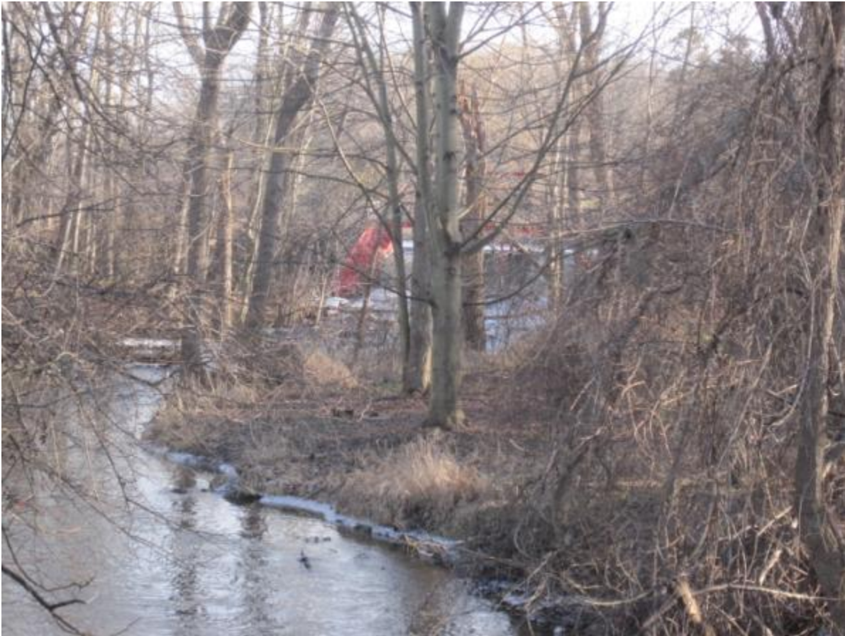
Mill dam looking north
