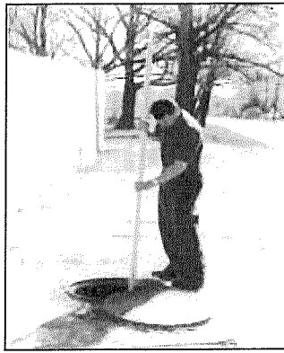
Figure 1. Measuring sediment in swirl chamber using stadia rod. Inspections are performed from the surface through the manhole access cover.
