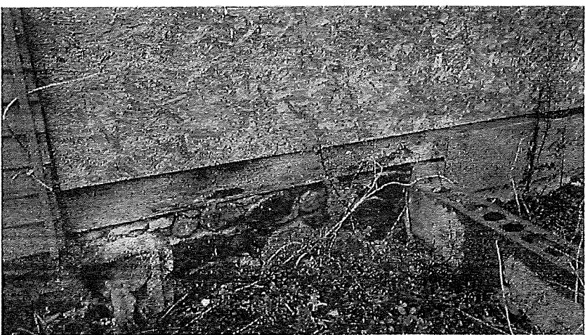
Sill and Foundation at South
