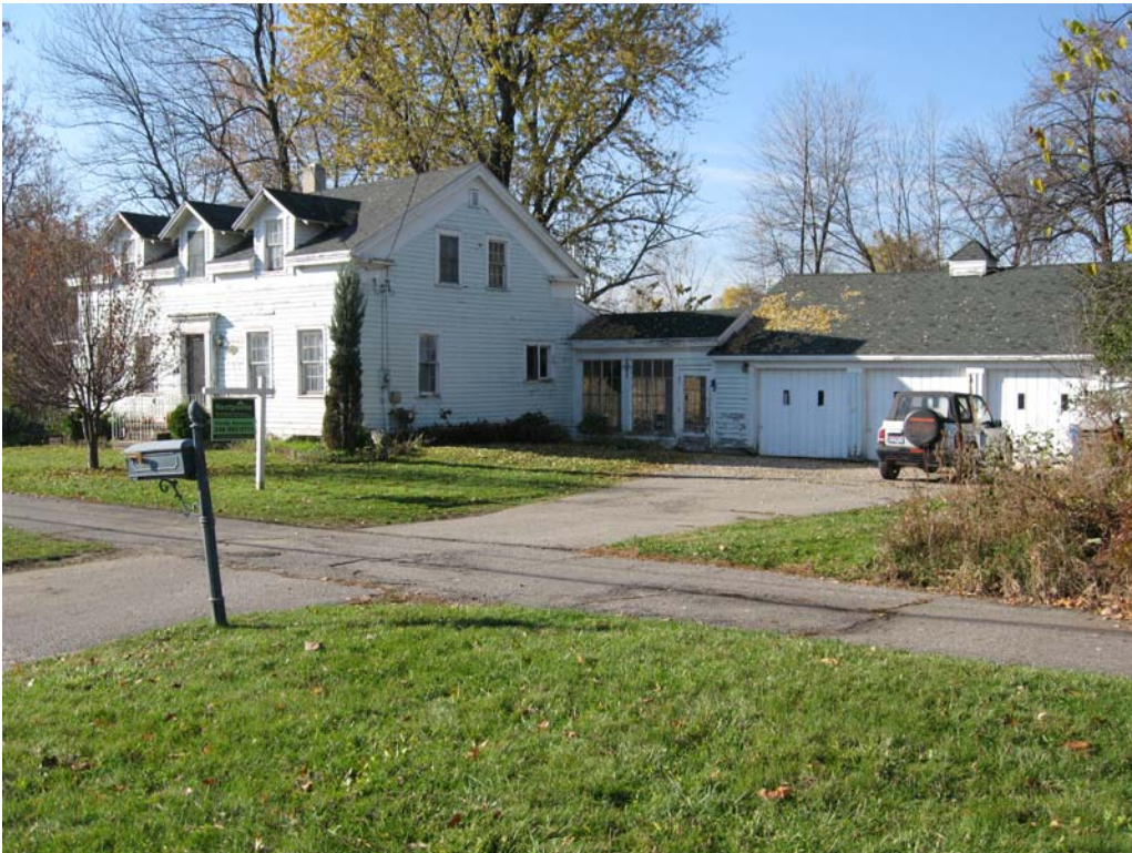
Photo 2. Williams S. Adams House, looking southwest
