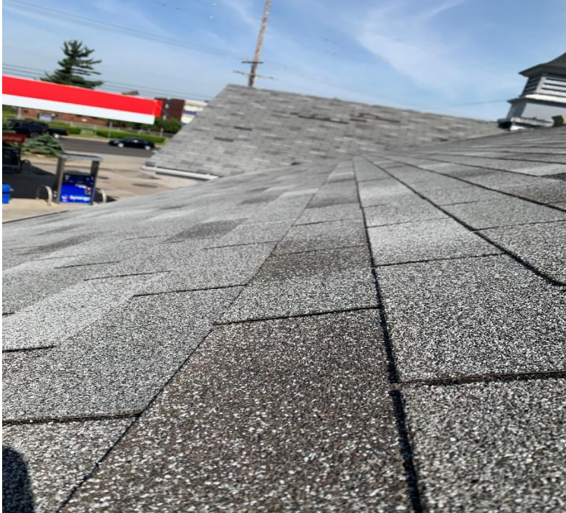
View of Roofing Shingles and Underlayment (HA8)
