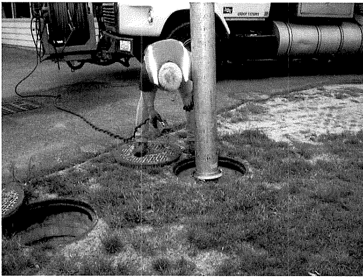
A Cascade Separator unit can be easily cleaned in less than 30 minutes.
