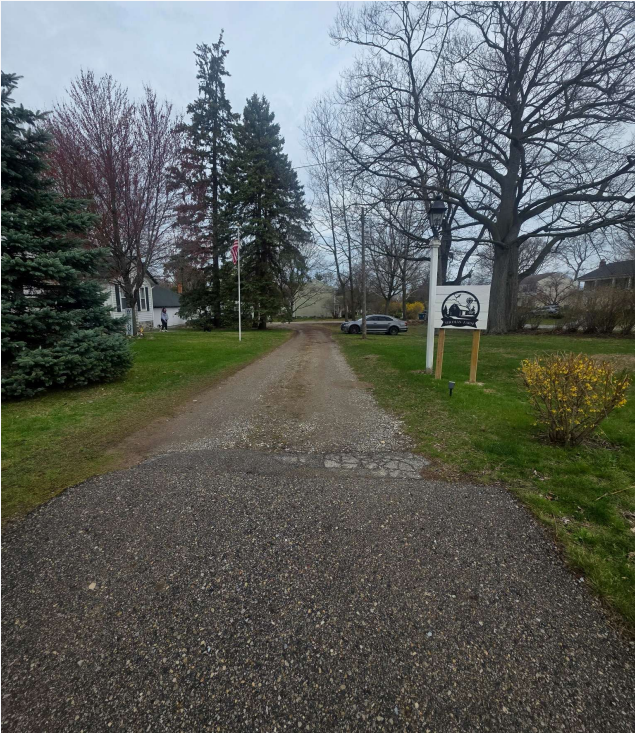
Entrance from Tienken RD
