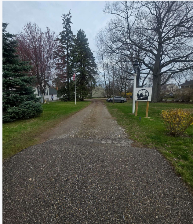
Entrance transition from asphalt to gravel
