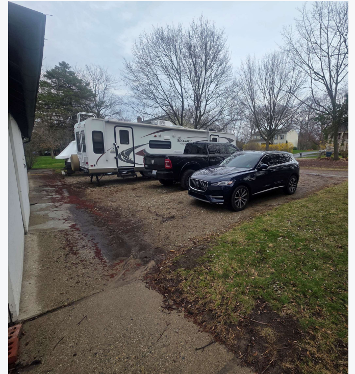
Entrance transition from asphalt to gravel
