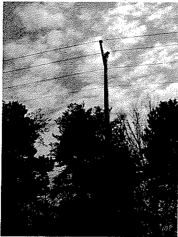
P15. Utility pole (X5, N3 on site map)
