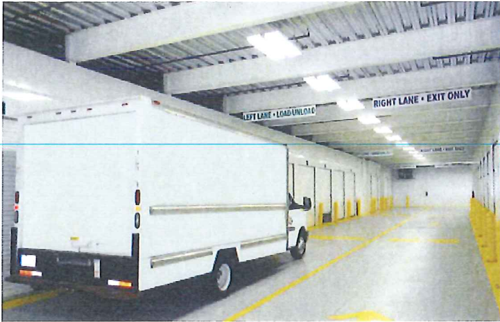
Covered Loading Areas
