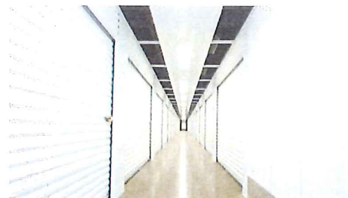
Motion Detected Lighting
