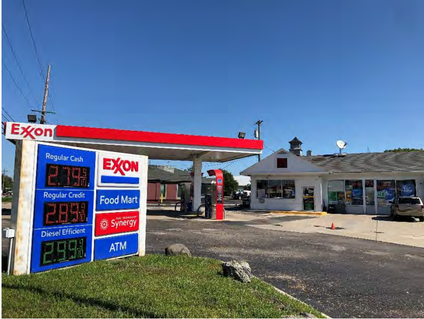
Overall view of the 975 South Rochester Road.
