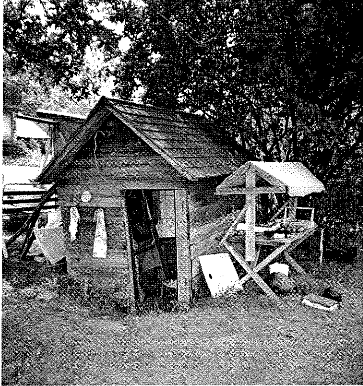
Photo 5. Well house, looking southwest.
