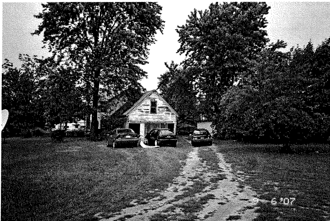
Photo 7. Loren Frank House garage, looking northeast. Milk house visible on right.
