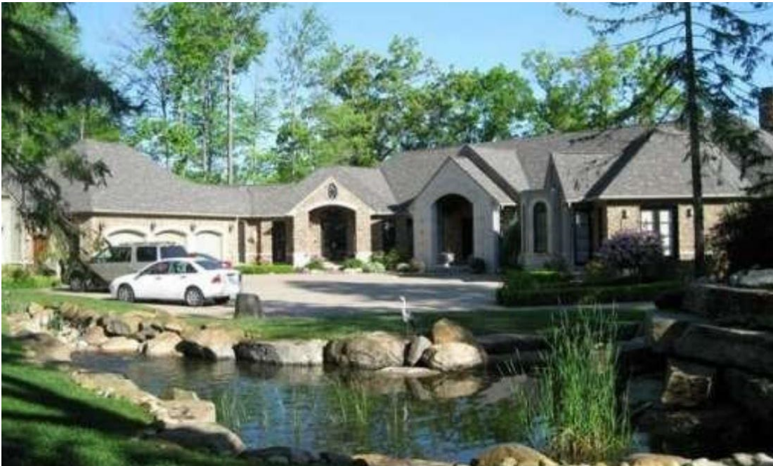
1965 Washington Road, c. 2005, non-contributing, Assessor photo, unknown date
