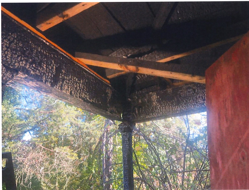
Alternate view of front porch at northeast corner.
