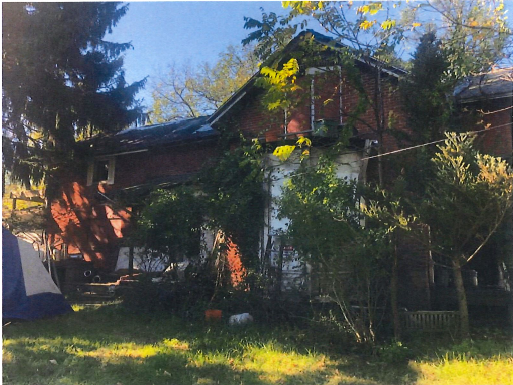
East side of subject structure looking southwest.
