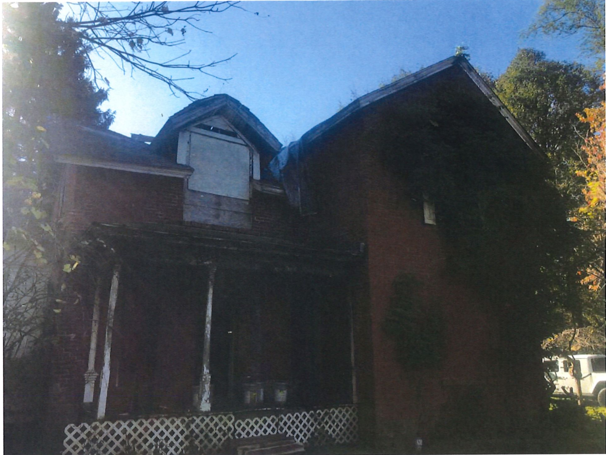
Front of subject structure looking south.
