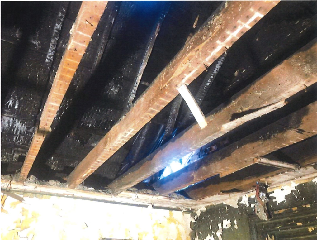
Roof and ceiling framing over second floor.
