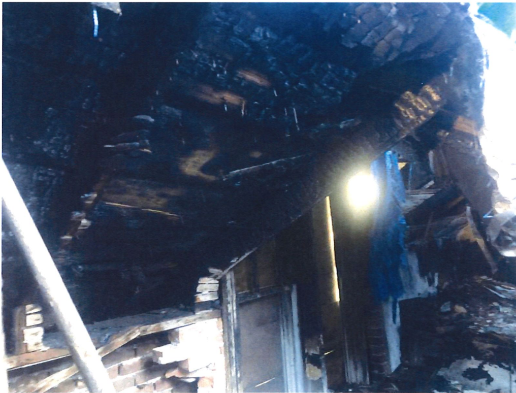
Alternate photograph of roof and ceiling framing over second floor.
