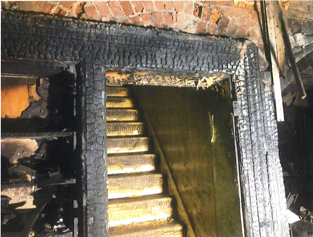
Access stair to second floor with limited head room.
