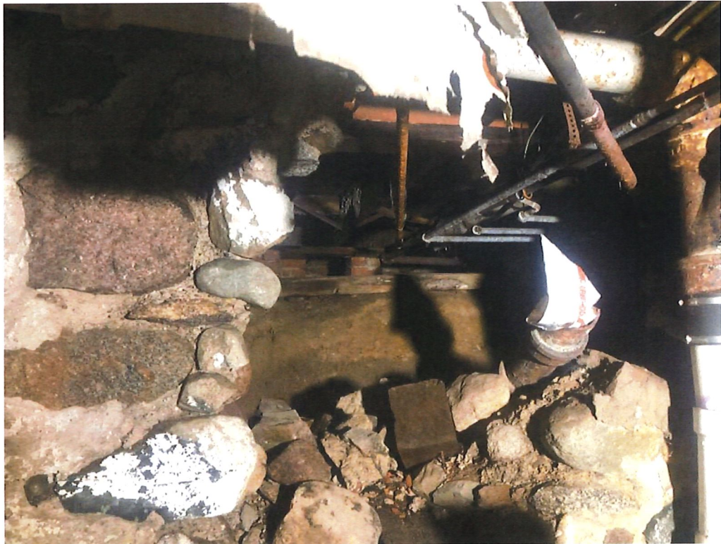
View into crawl space.
