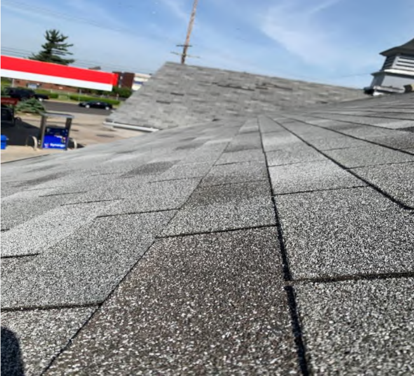
View of Roofing Shingles and Underlayment (HA8)
