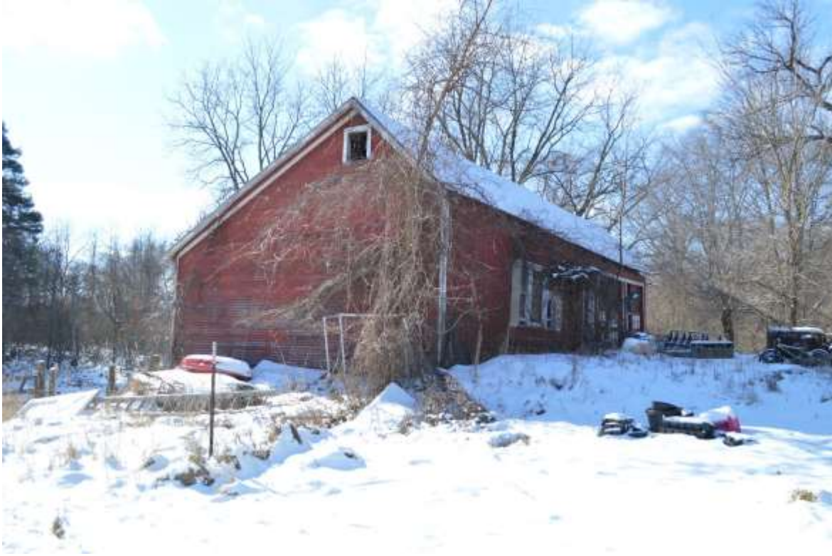
7-Looking southwest at barn north and east elevations, January 2021
