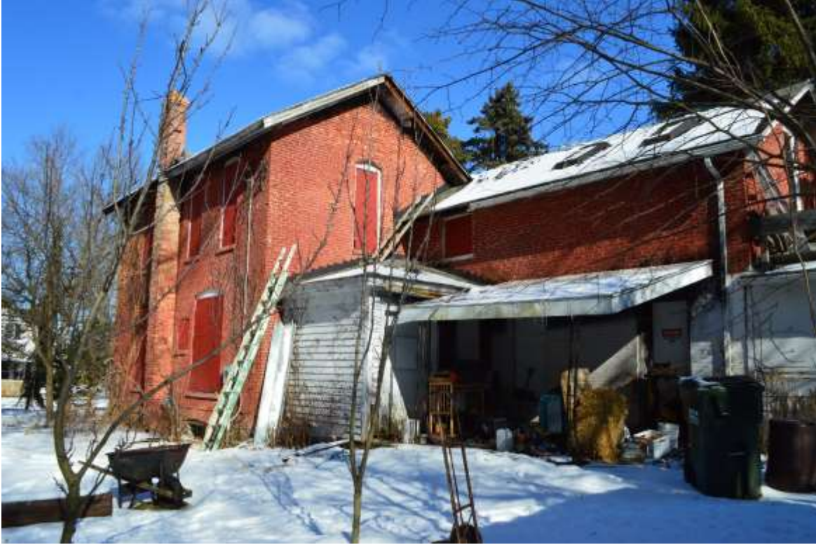
5-Looking northeast at west side and rear of house, January 2021
