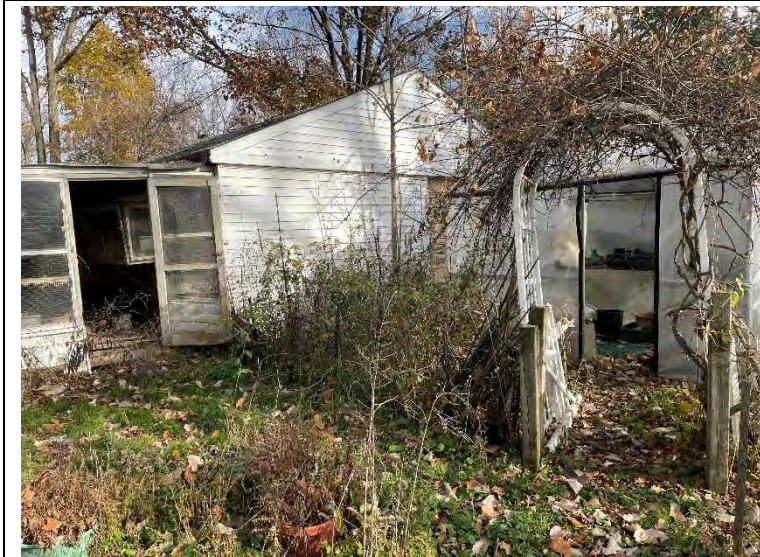
Photo 8. View of shed and green house
