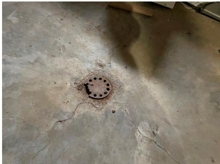
Photo 15. Drain in basement
