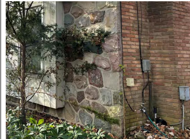
Photo 3. Possible fill ports for the AST to the left of the chimney
