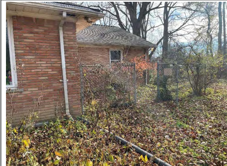
Photo 5. West side of house, facing southeast
