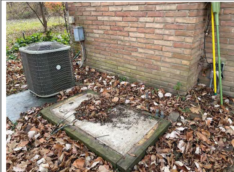
Photo 2. HVAC unit and concrete pad for prior Generac generator on North side of house
