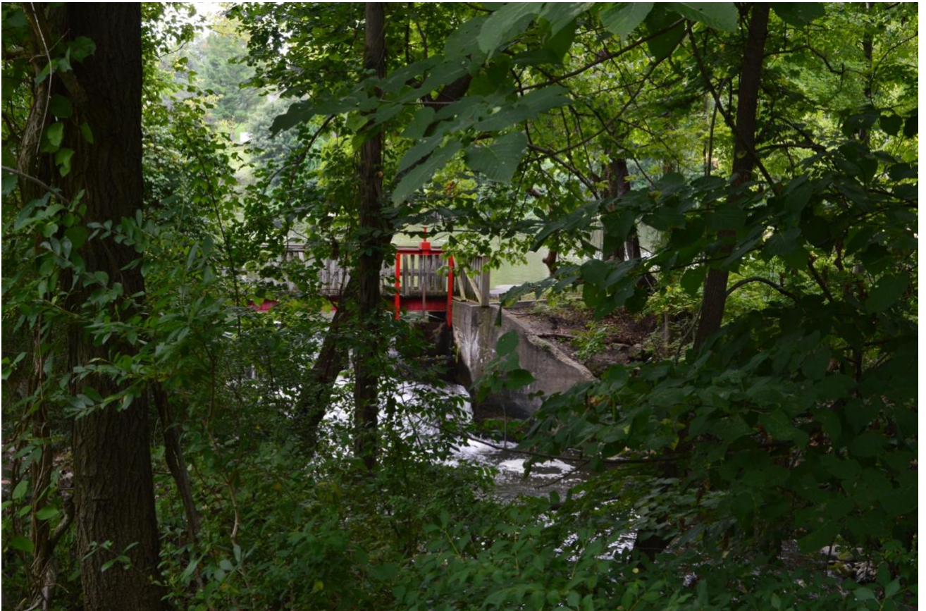
Photo 6 Looking north at dam with mill pond beyond
