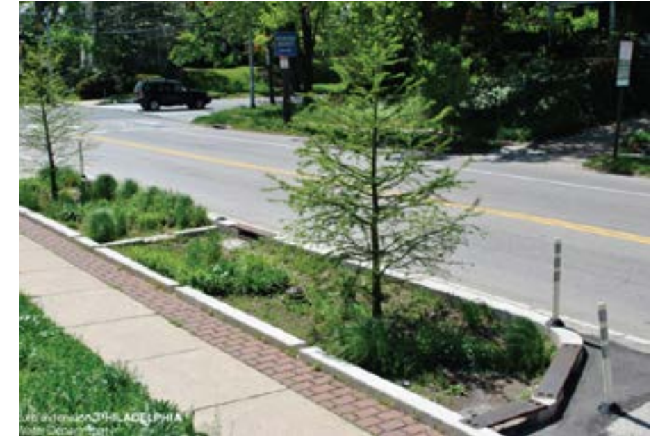
Curb extension GSI in Philadelphia, PA.
