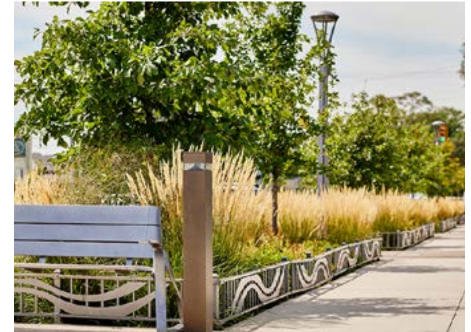
Tree box bioretention planters in the Brooklands District.
