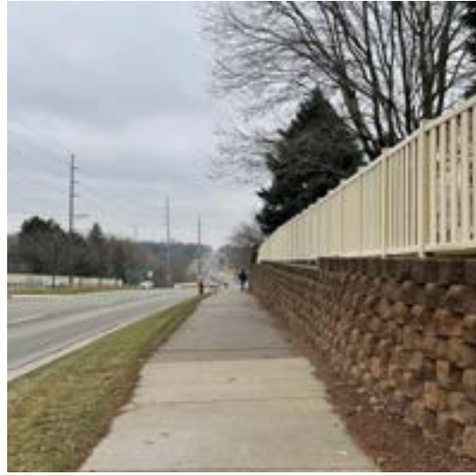
Vinyl Fencing and Retaining Wall
