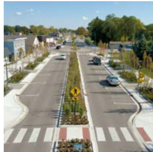
Crosswalks, mid-block crossings, abundant median and street landscaping
