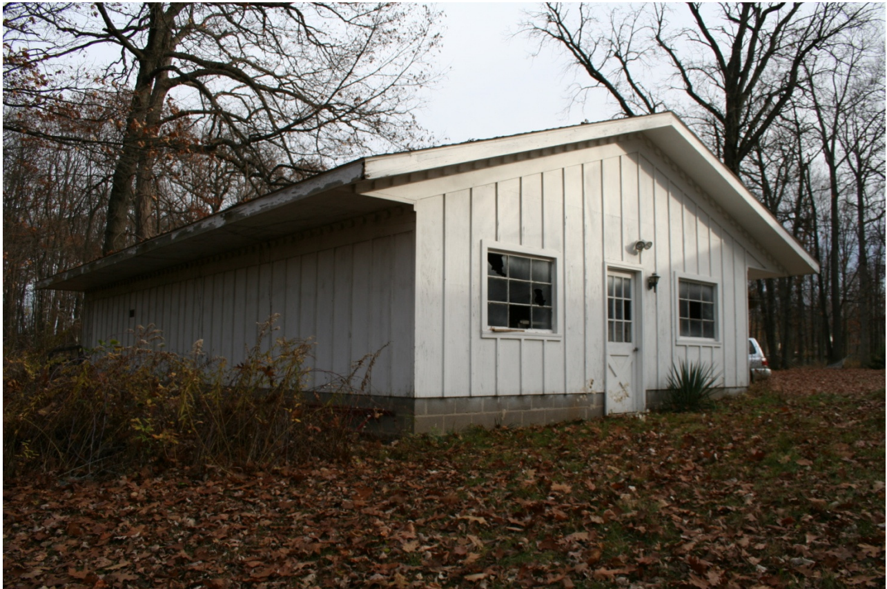
Photo 6 2371 South Livernois, garage, north and west elevations looking southeast, November, 2009
