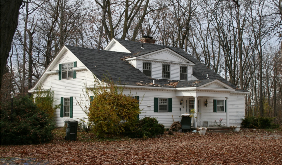
Photo 2 2371 South Livernois, south and east elevations looking northwest, November, 2009
