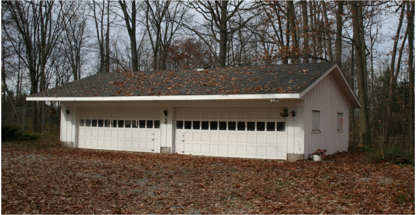
Photo 5 2371 South Livernois, garage, south and east elevations, looking northwest, November, 2009
