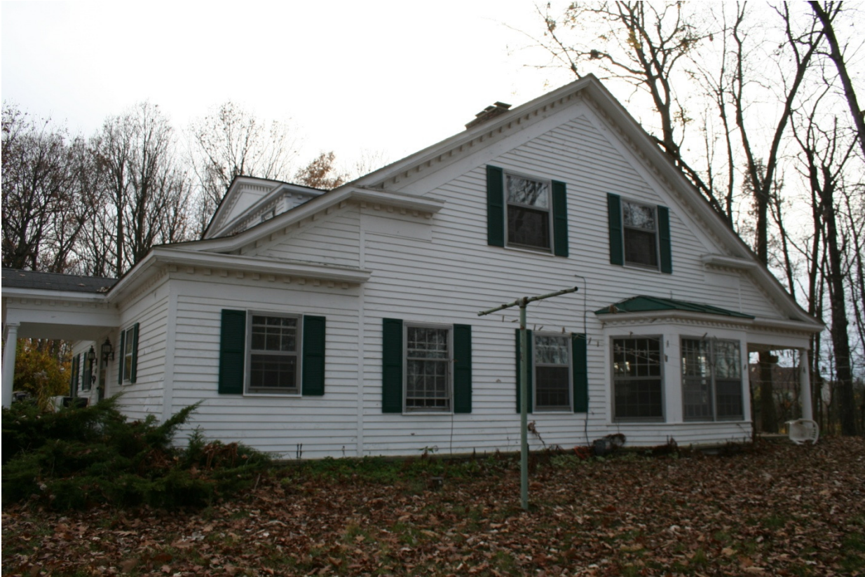
Photo 3 2371 South Livernois, north elevation looking southwest, November, 2009
