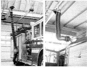
The MagnaTrack HS is designed to serve emergency stations with a high frequency of runs. The track system serves one vehicle at a time. The balancer has a constant liftning power.
