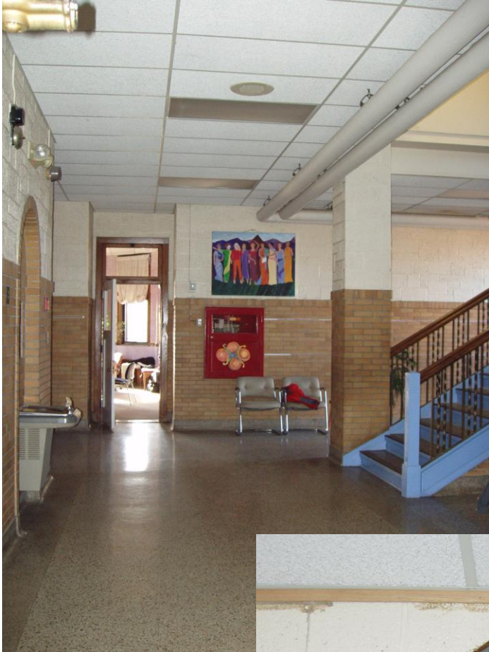
Photo 6: Main first floor corridor in 1929 building.
