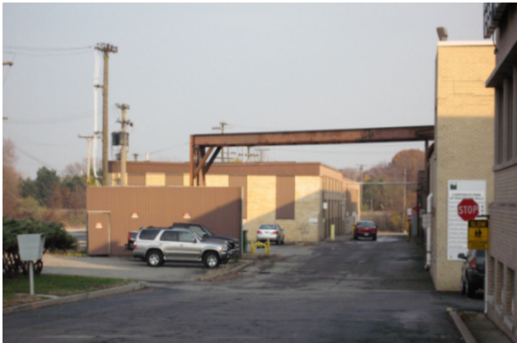
Photo 5. Utility structure (H) in front; factory building (E) in rear, looking northeast. Photo by Jane Busch, November 2008.
