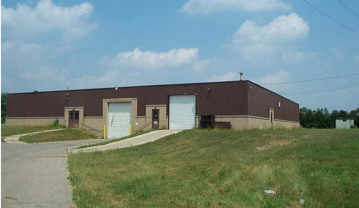
Photo 6. Factory building (F); utility structure (K) in background, looking northeast. Photo by Burke Jenkins, Hamilton Anderson Associates, May 2002.
