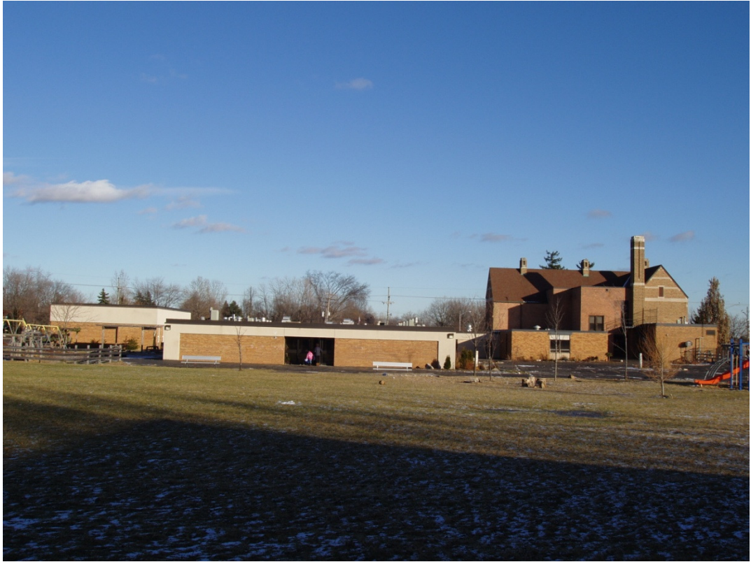
Photo 3: Stiles School, west elevation, 1958 & 1963 additions on left (not in district).
