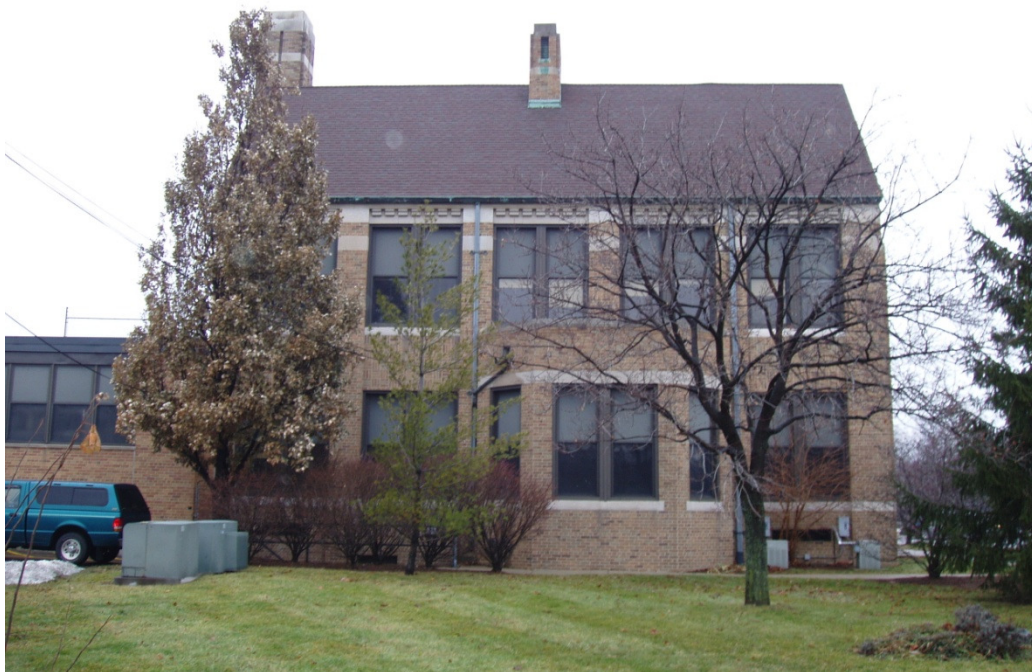
Photo 2: South elevation, note first floor bay for kindergarten room.
