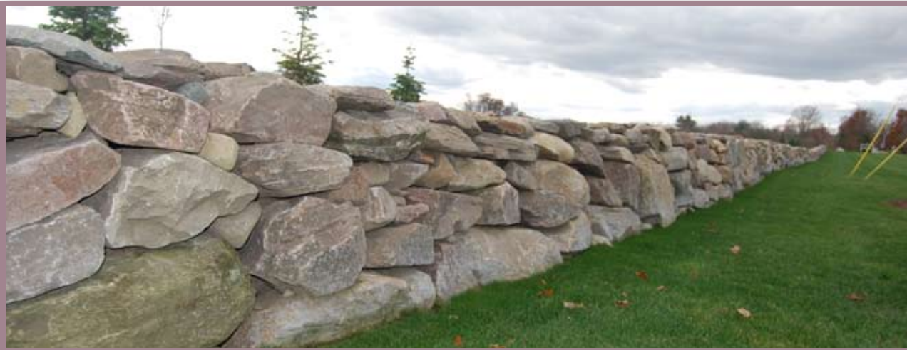
▼ Example of a loose laid stone wall. National Cemetery in Holly, MI.
