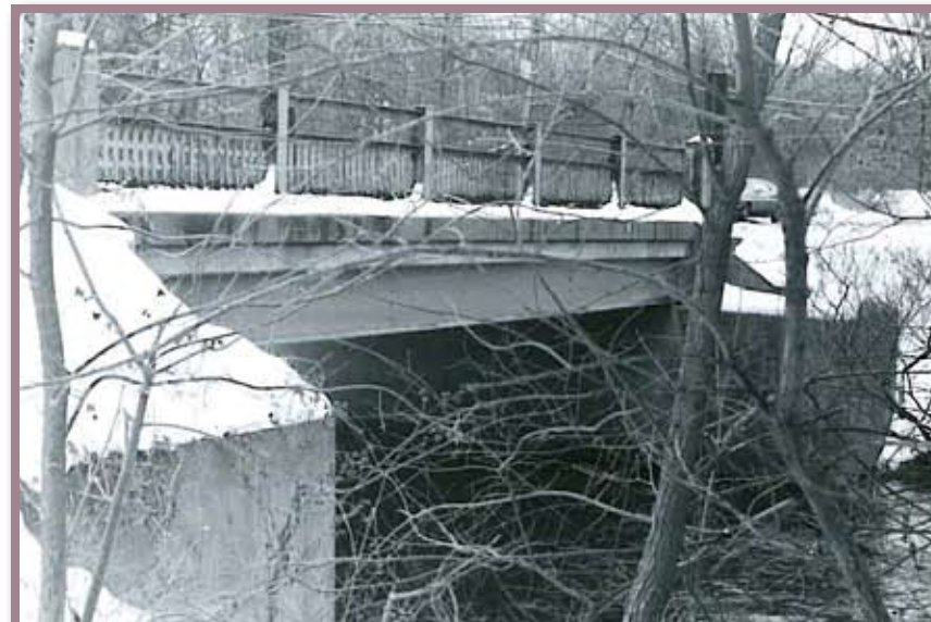
Stoney Creek Bridge circa 1978 ▶
