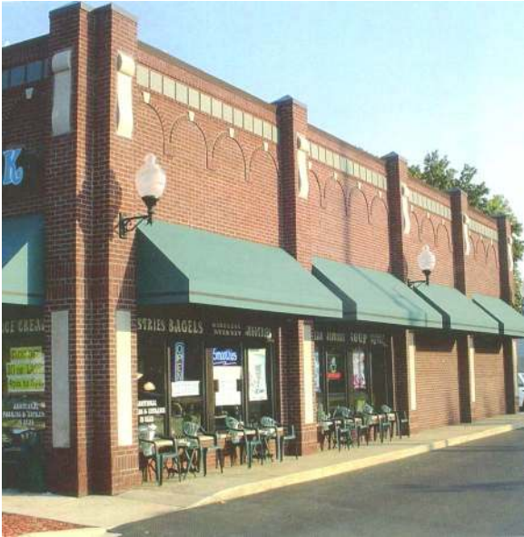
Figure 7.5 – Articulated Upper Facade
