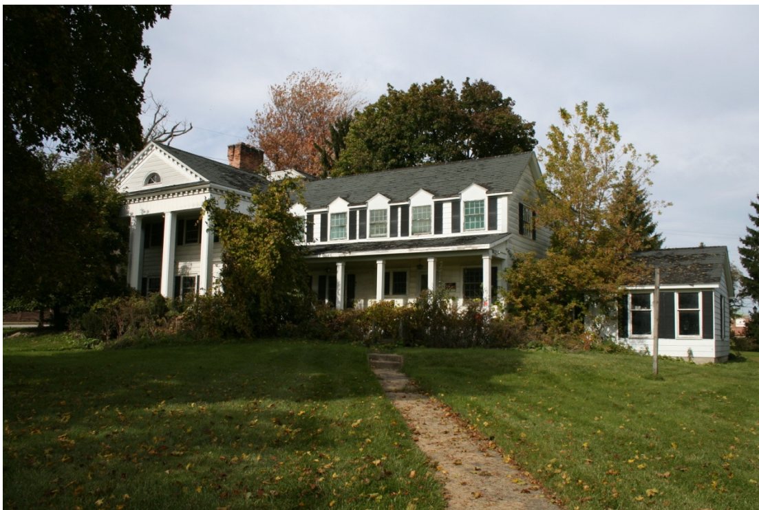
South elevation looking northwest, October, 2009
