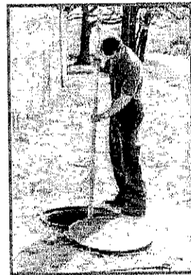
Sediment inspection using a stadia rod
