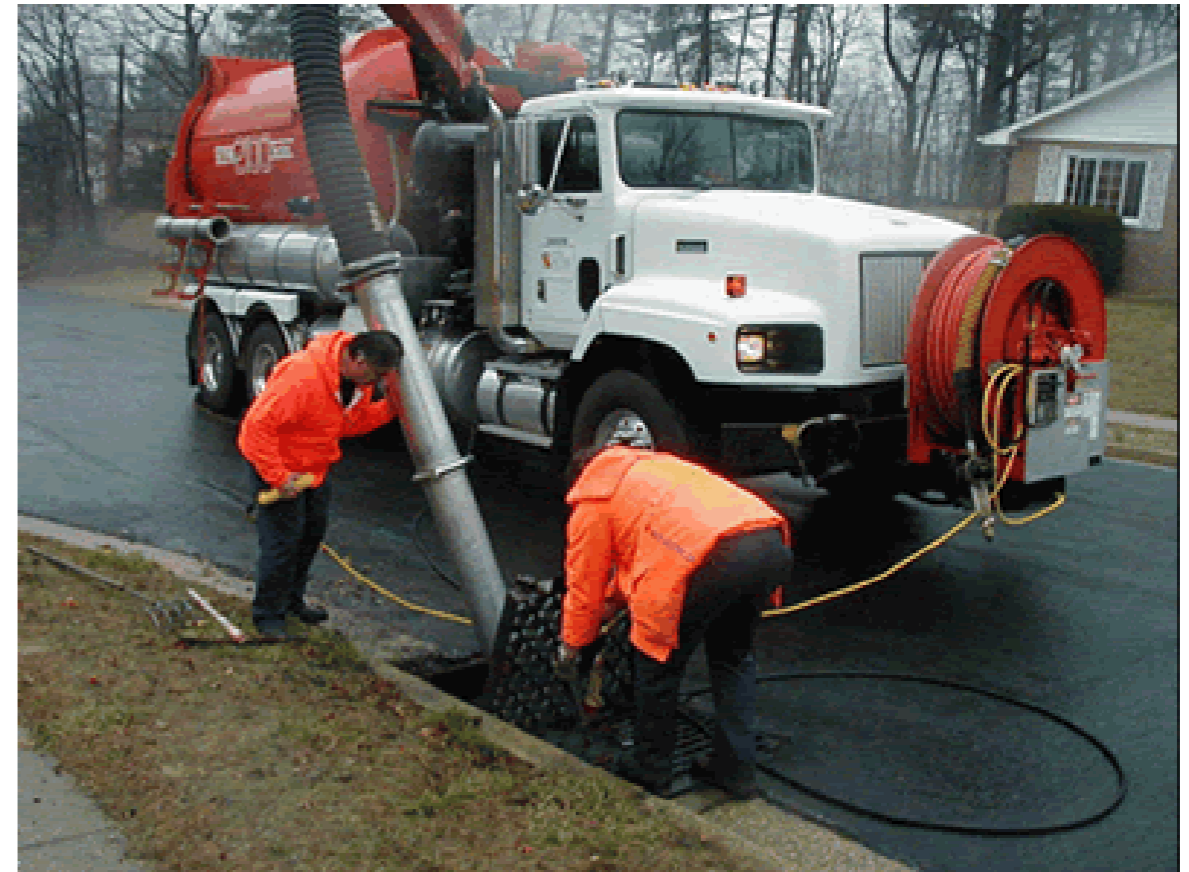
Catch Basin Cleaning
