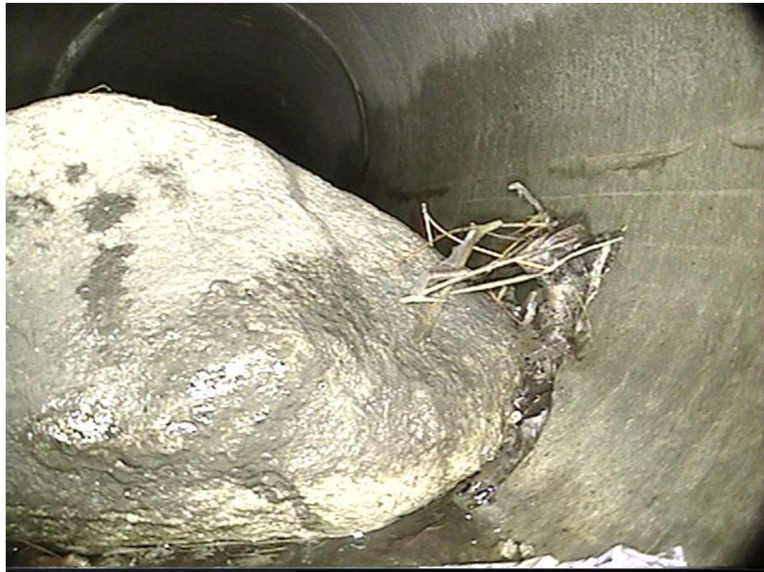
Sewer Clean to Remove Obstructions
