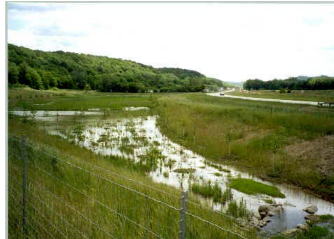
Stormwater Treatment Wetland
