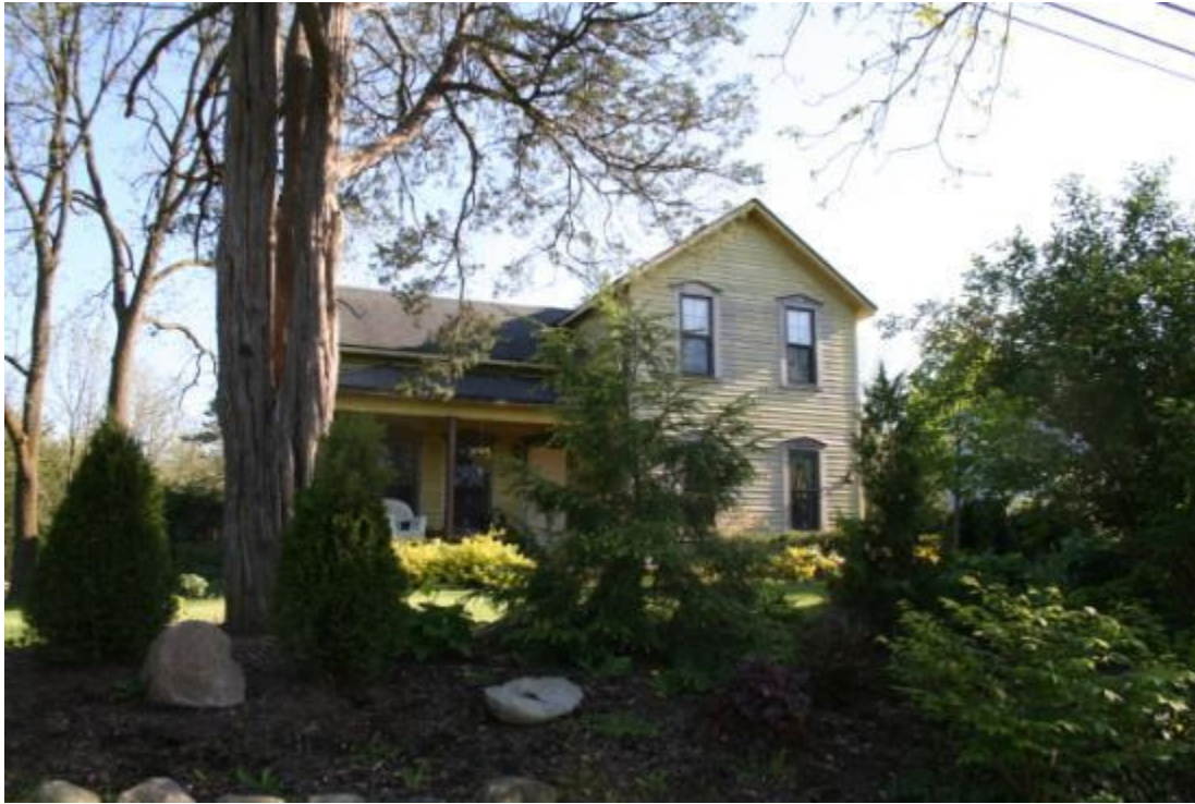
Looking southwest at 1631 W. Avon Road, May 2012
